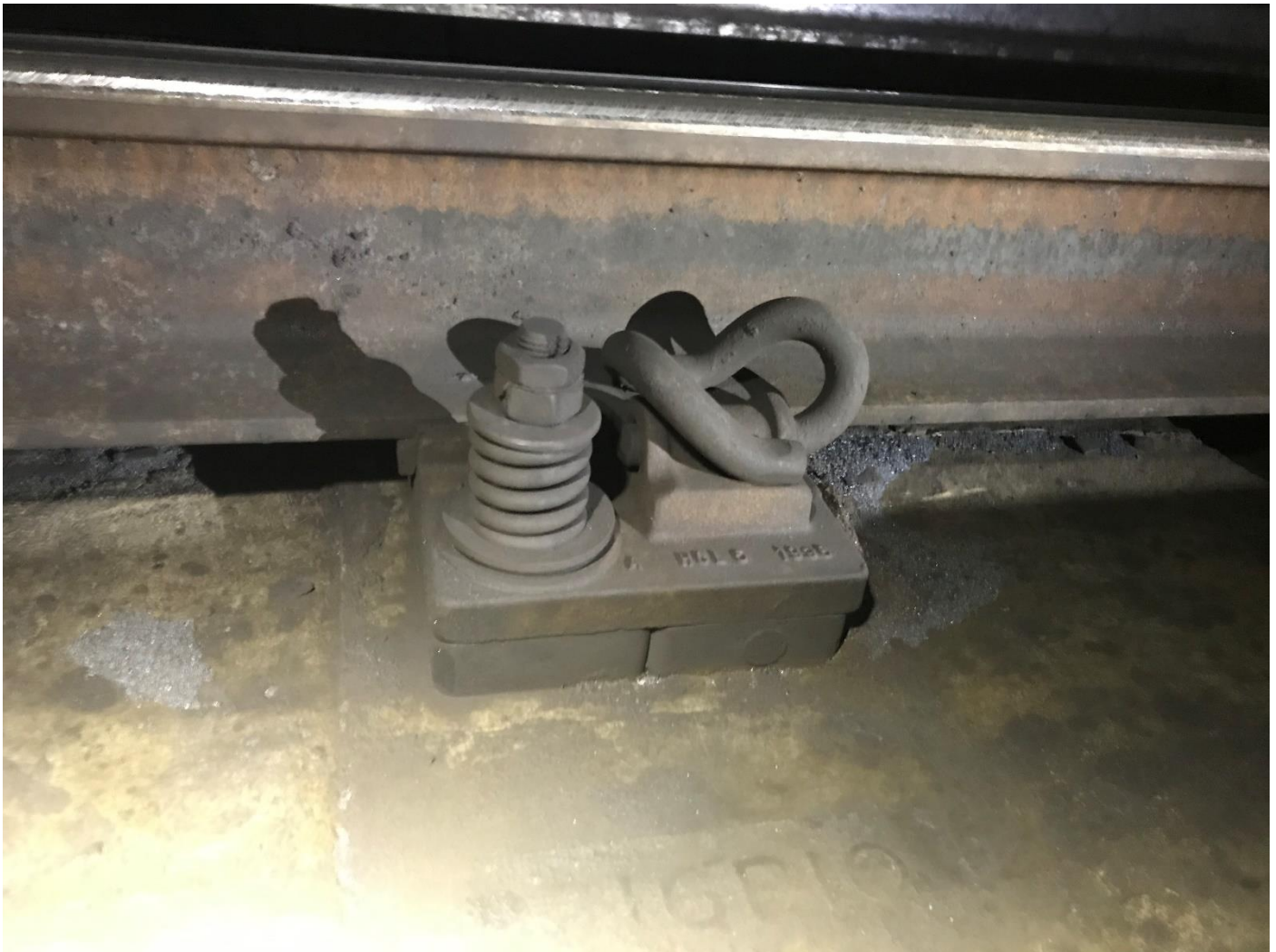
Figure 2 – Resilient track fixing on the eastbound Jubilee line, right-hand rail
